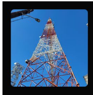
Tower and Antenna
